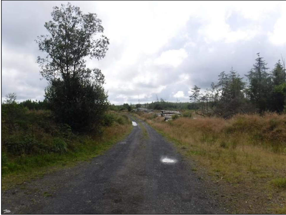
Photo 1 Example of existing founded track on site
